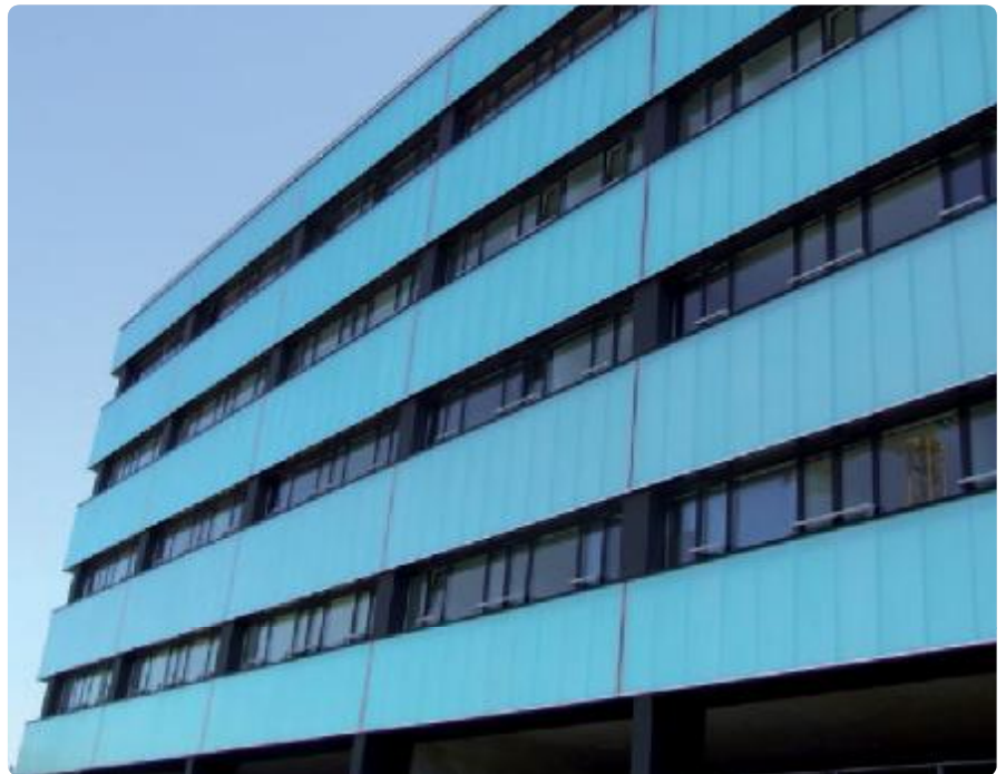
TRANSLUCENT CURTAIN WALLS Realization vertical translucent curtain walls
